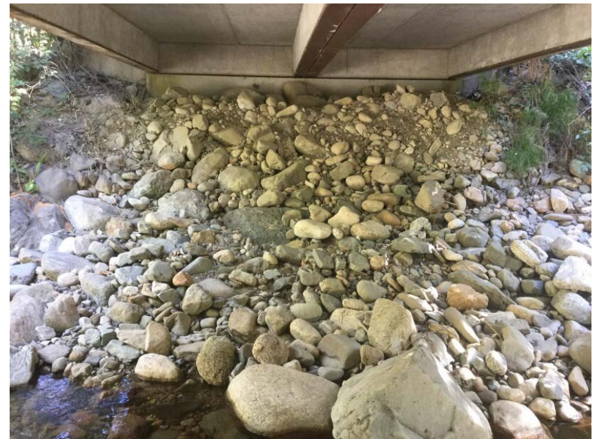
Right Bank Abutment when facing downstream
