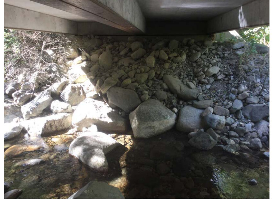
Left Bank Abutment when facing downstream
