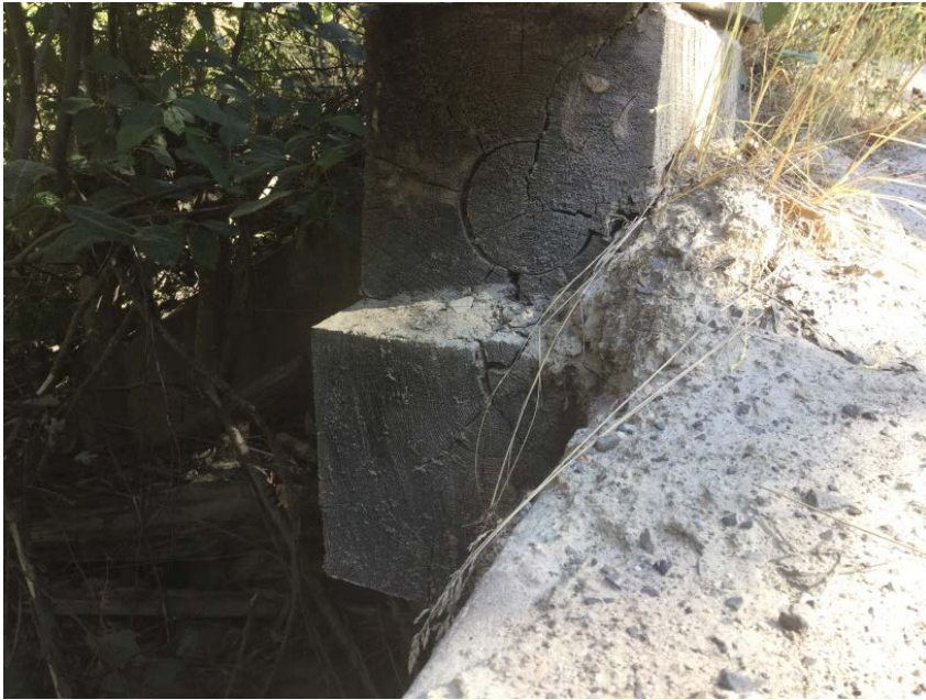
Riser and block condition - typical
